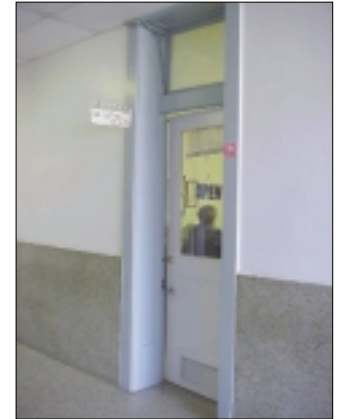
Detail of terrazzo, Room 108
