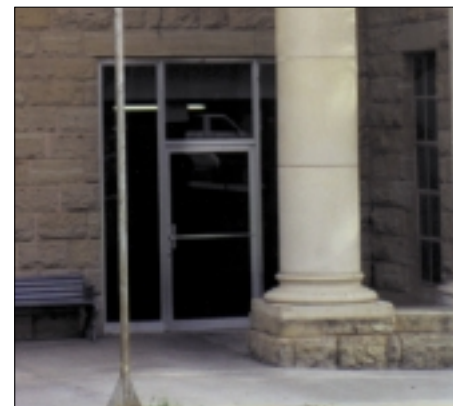
Detail of front porch (west elevation)
