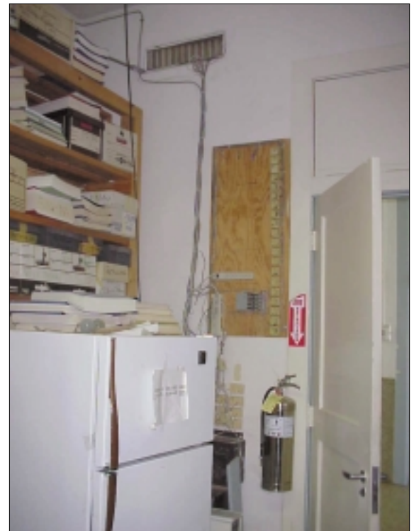
Detail of storage, Room 104
