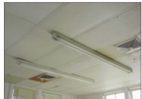
Ceiling in Room 201
