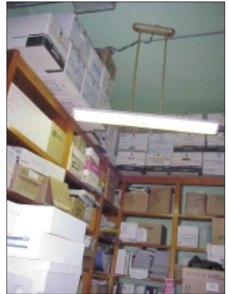
View into storage, Room 110
