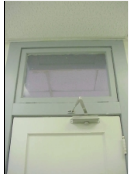
Detail of door, men's restroom, Room 113
