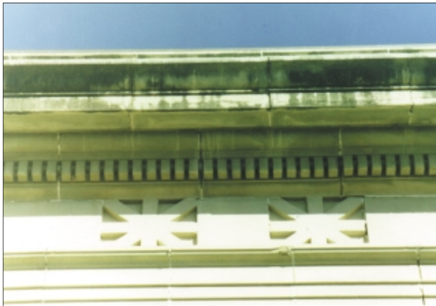
South elevation, east end of cornice
