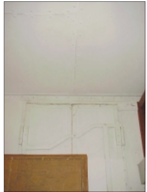
Detail of county vault door, Room 103
